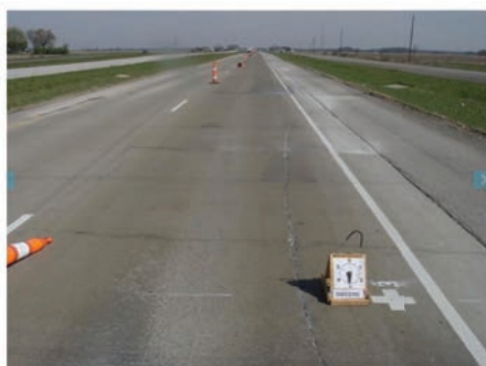
Figure 29. Longitudinal cracking near the shoulder in Ohio-0206 section (September 12, 2006).
